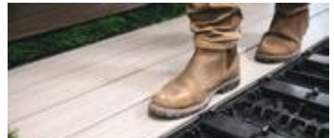
Step 3. Step down to snap boards in
