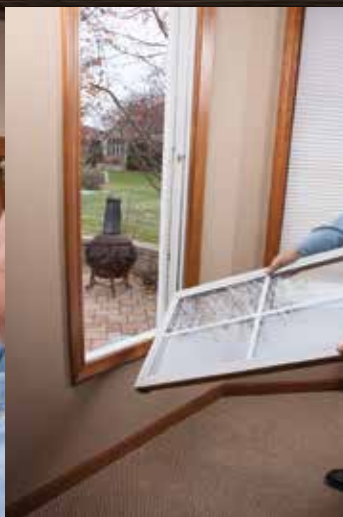
Step 3 Install new sash.
