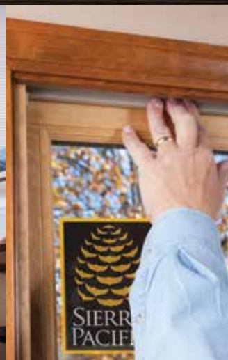
Step 4 Install new head weatherstripping.
